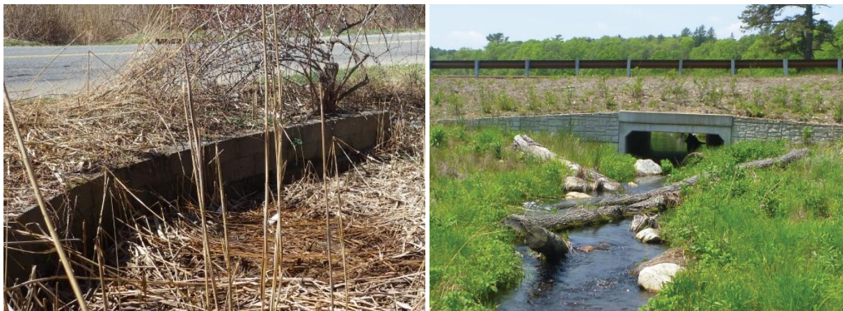
Left: Existing non-functional stream culvert on East Branch of Mud Creek at Gazzola Drive. Right: Constructed eco-friendly box culvert and stream channel under Long Pond Road, Eel River (MA).
